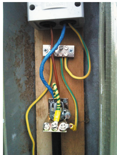
Example of CET 003 being used with EB42 earth block feeding isolator with plastic gland plate
