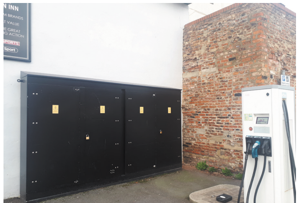
EV Distribution Pillar for Highways England supporting standard and rapid charging.
