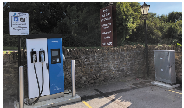
EV Distribution Pillar for Highways England supporting standard and rapid charging.
